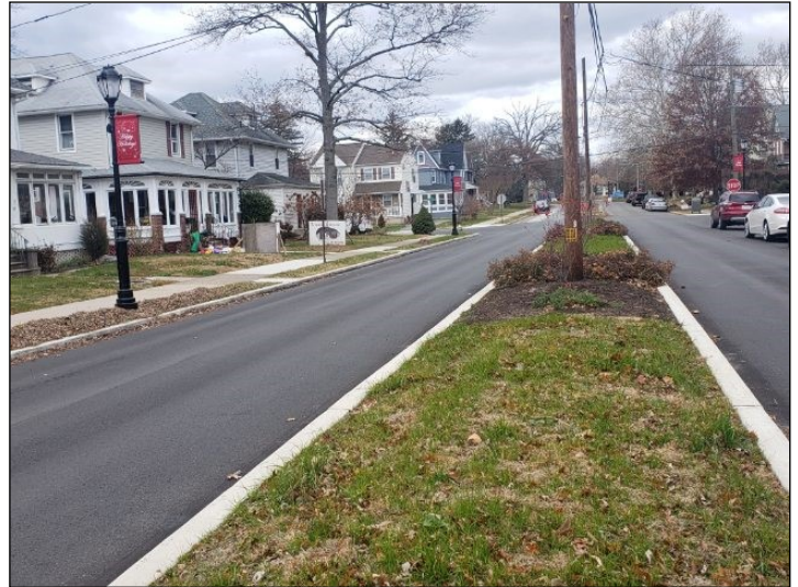
Prospect Avenue streetscape improvements included street resurfacing and the installation of median curbs, decorative lighting and banners.
