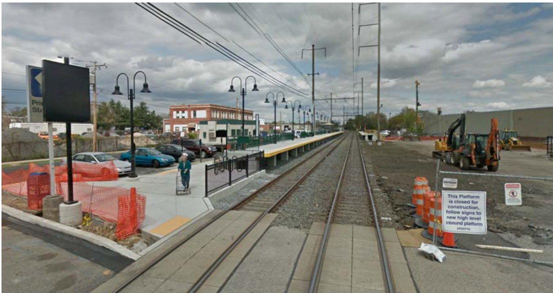
Construction of ADA accessible platforms at Primos Station on the Media-Elwyn Line. Image source: Google street view
