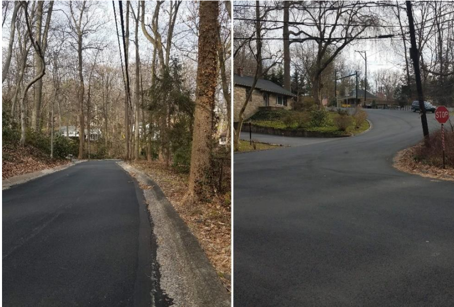
Very steep sections of Beechwood Road (left) and Pine Ridge Road (C5)
