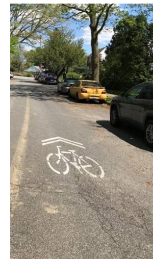
Typical Sharrow Street marking in Media Borough
