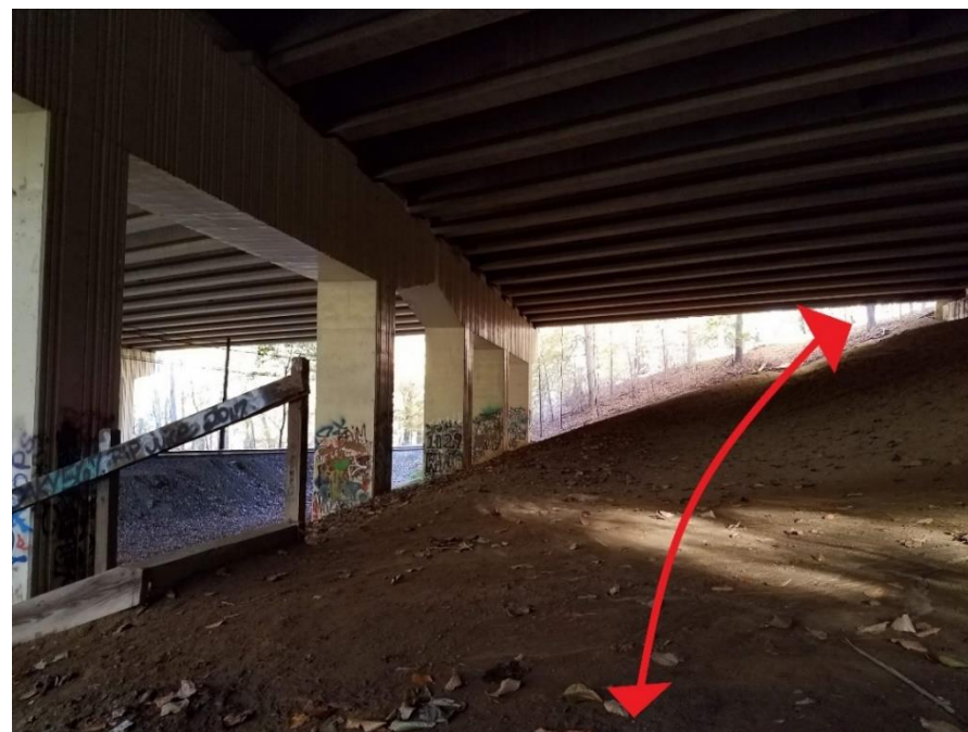
Location recommended for trail Segment J under I-476 (view east with SEPTA Trolley on left)
