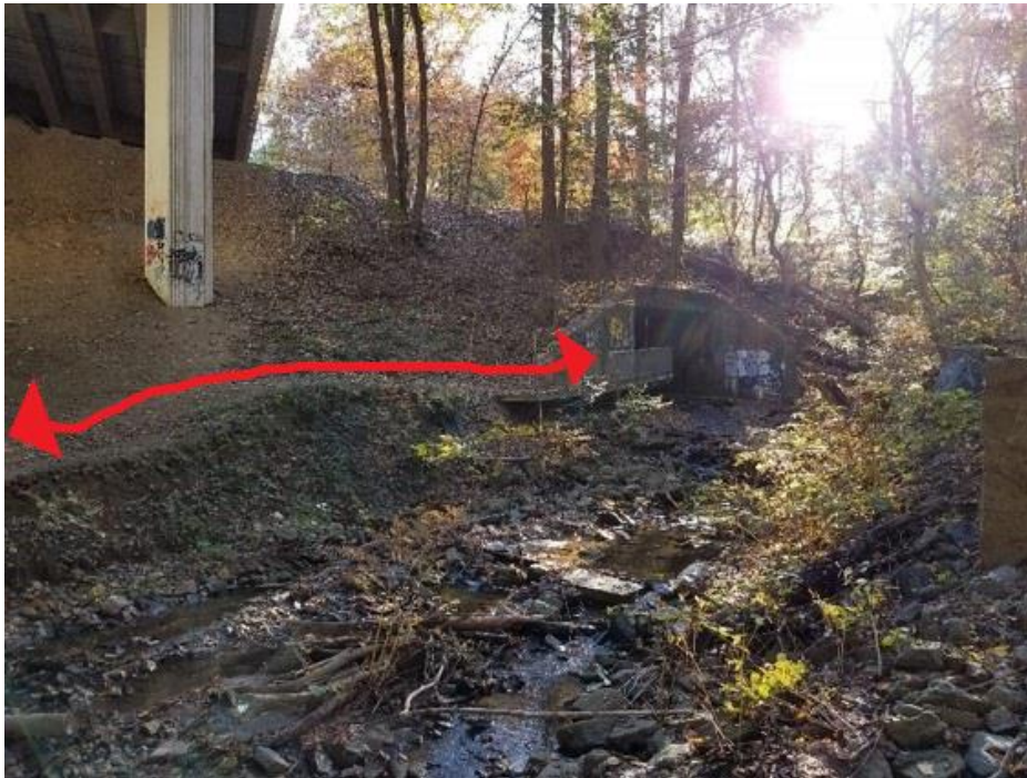
Segment K Trail location under I-476 leading to North side of the Culvert Walkway under SEPTA Trolley.
