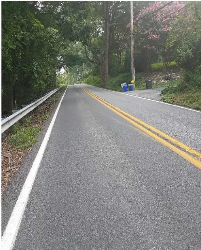
Kirk Lane, steep with no shoulders (A5)
