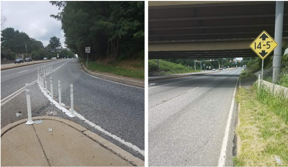
Views west on Baltimore Pike at I-476 off-ramp next to Smedley Park (left) and under-476 (right) (D3)
