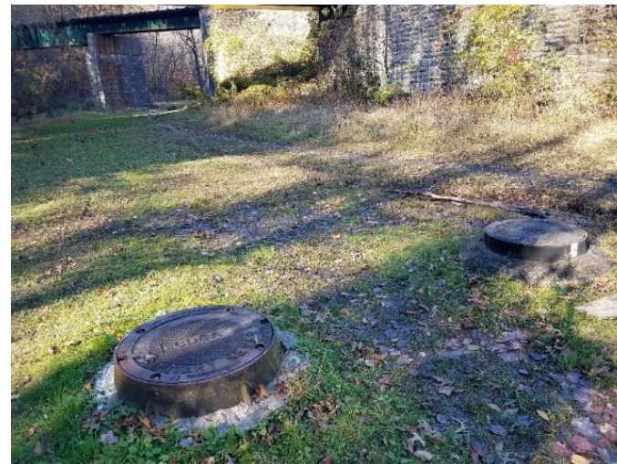
Along the CDCA sewer line right-of-way on the east side of Crum Creek (D7)
