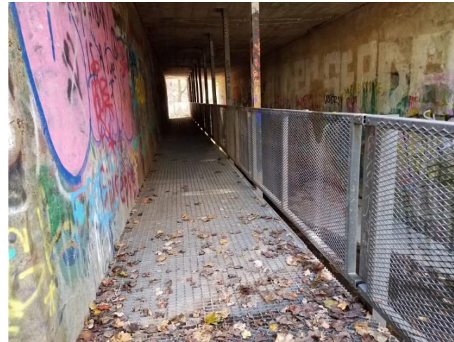
Culvert with walkway under SEPTA Trolley (D4)
