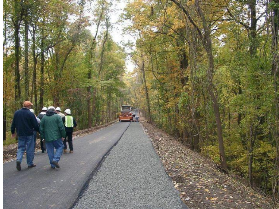
Paving of a multi-use trail (Photo Credit: Friends of the Radnor Trail)
