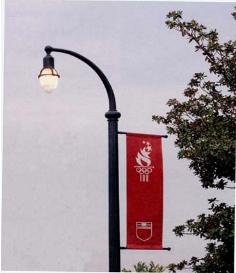
Holophane ("Atlanta") fixture; Highway height lighting can also be decorative.
