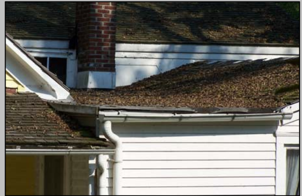
Gutter systems that are clogged with debris or bow will not function correctly and can lead to water pooling down the side of your house or seeping under roofing materials
