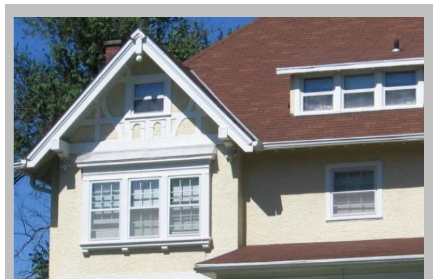
These exterior storm windows are perfectly fitted with the historic windows so that the meeting rail on the storm window aligns with that of the historic window. In addition, the trim color and scale is appropriate for the window openings
