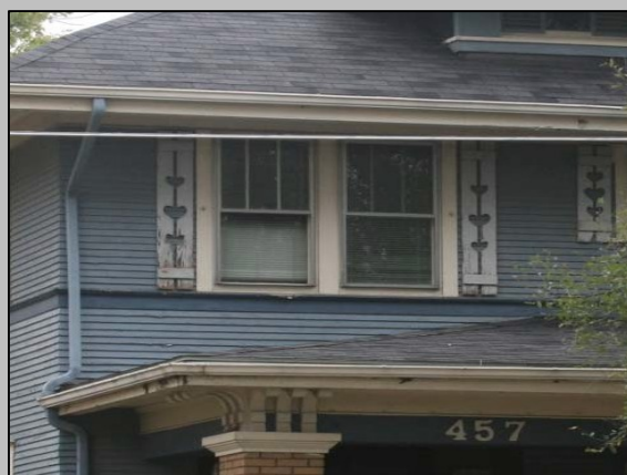
Shutters should only be installed where they were historically found. They should also be installed as a functional building element that covers the entire window opening, not simply as a decorative element as they are on this house.
