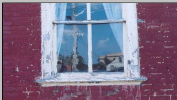
To ensure a long operating life, windows should be regularly maintained, and deterioration should be addressed before it compromises the structural stability and efficiency of the unit.
