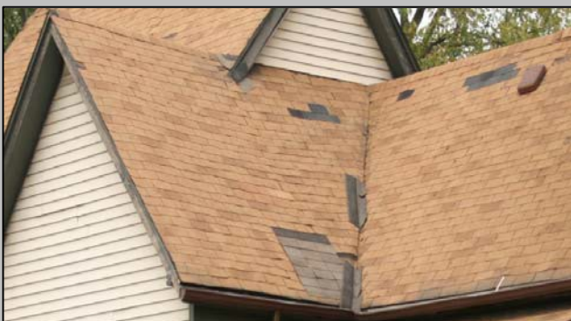
The roofing system is the house's first line of defense in deterring moisture infiltration, air infiltration, and pests. As such, the roof should be well maintained, and any damage should be immediately addressed so that it does not compromise the ability of the roofing system to function correctly.
