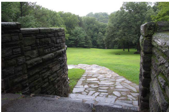
Figure 3-12: Stairs from overlook structure
