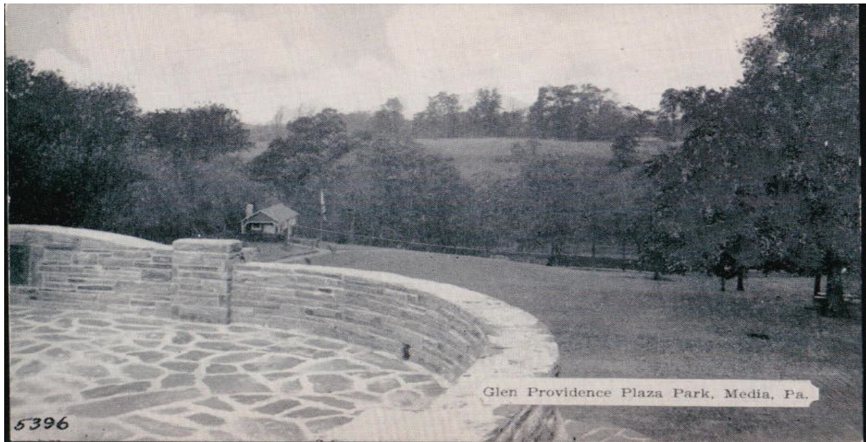
Figure 3-18: Overlook structure (date unknown)
