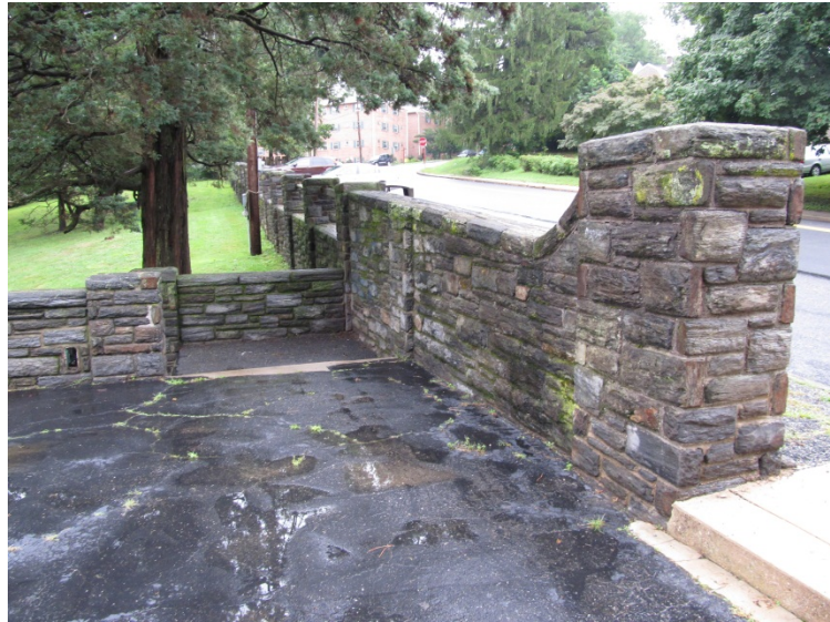
Figure 3-20: Overlook structure entrance
