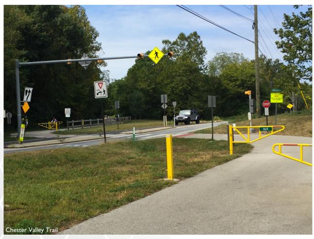
Trails should be designed to meet roadways at right angles to provide adequate sightlines at the intersection (below).
