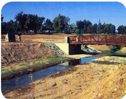
The reconfiguration of stream banks can increase the capacity of the waterway and lower the water elevation during flood events.
