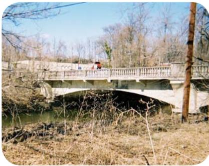
The low arches of the Kerlin Street bridge often collect debris and obstructs the flow of water.
