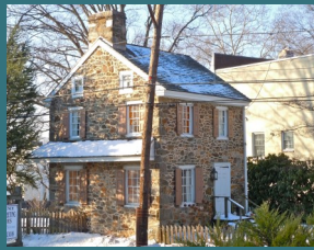
The Minshall House (1750) Style: Colonial Vernacular
