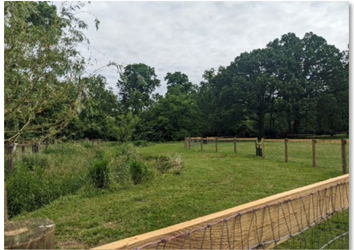
After streambank fencing (Edgmont Township)
