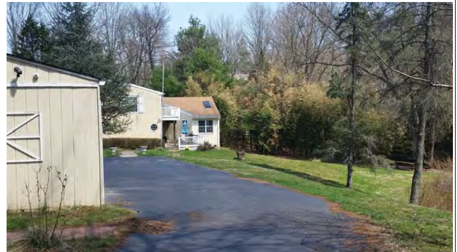
Caption: West Elevation & Garage; Camera Direction E
