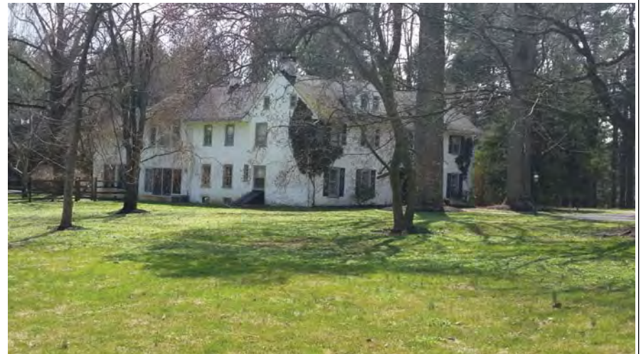
Caption: East Elevation, Camera Direction: SW
