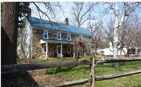
373 Glen Mills Road, Thornbury
