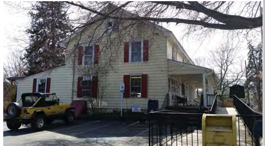
Caption: East Elevation; Camera Direction: W
